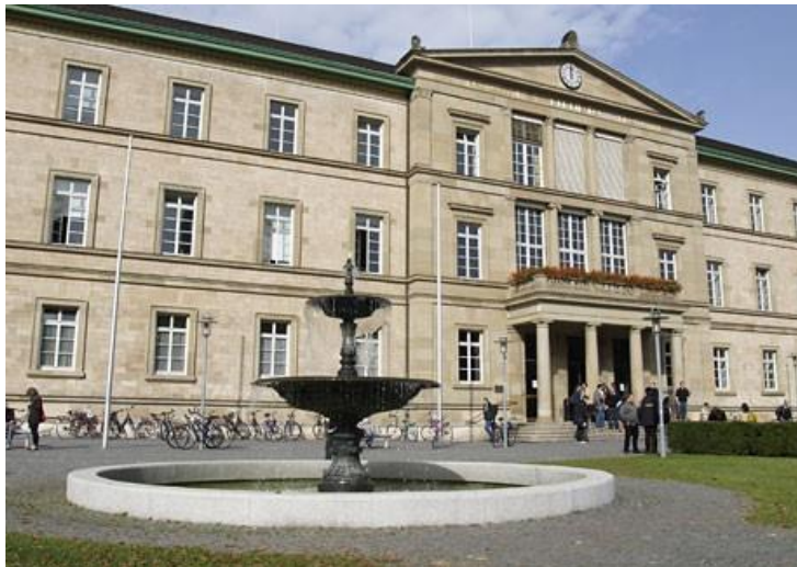
Neue Aula, Tübingen Centre
